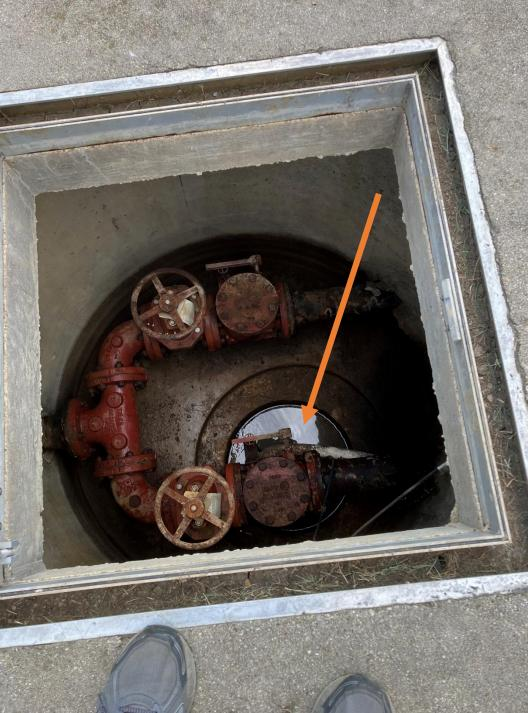
The Gate Valves at a Lift Station Should be **Operated to Full Closed and then Back to Full Open, at Least Two Times a Year.** When the Valve is at Full Open, Close Valve ¼ Turn to Keep the Valve Off of the Seat/Stop. ( If You Don't Use it, You Lose it ) Working on Check Valves in Not a Pleasant Job if the Gate Valves will not Close.
