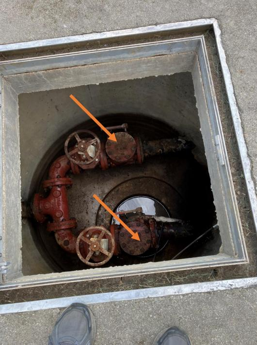
If The Valve Pit has a Sump Pump, It should be Tested on a Quarterly Basis, unless it appears that It is Not Working. Make Sure that the Float Switch is Moving Freely and does Not hang Up. Water Level should be in the Sump if it is Working Correctly. You Can Test Operation with a 5 Gallon Bucket of Water.
